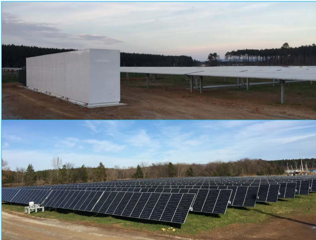
A 1 MW / 2 megawatt-hour battery storage system, coupled with a 10 MW, on-site solar array at Redstone Arsenal, AL
