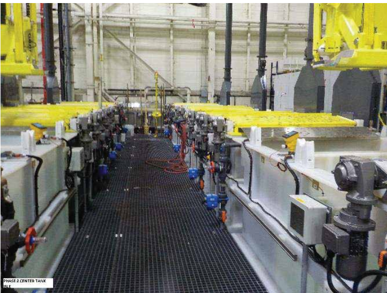
Rock Island Arsenal, Illinois - Joint Manufacturing Technology Center Modernization (ESPC)
