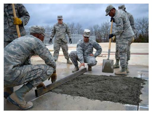
Figure C.1: Soldiers learning to repair airfield pavement (https://www.army.mil/article/164389/course\_lays\_foundation\_for\_airfield\_pavement\_management)
