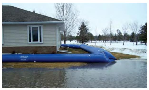
Figure C.6: Water-filled temporary barrier. The barrier shown in this figure is 2 ft high (FEMA 2014, Figure 8-4)
