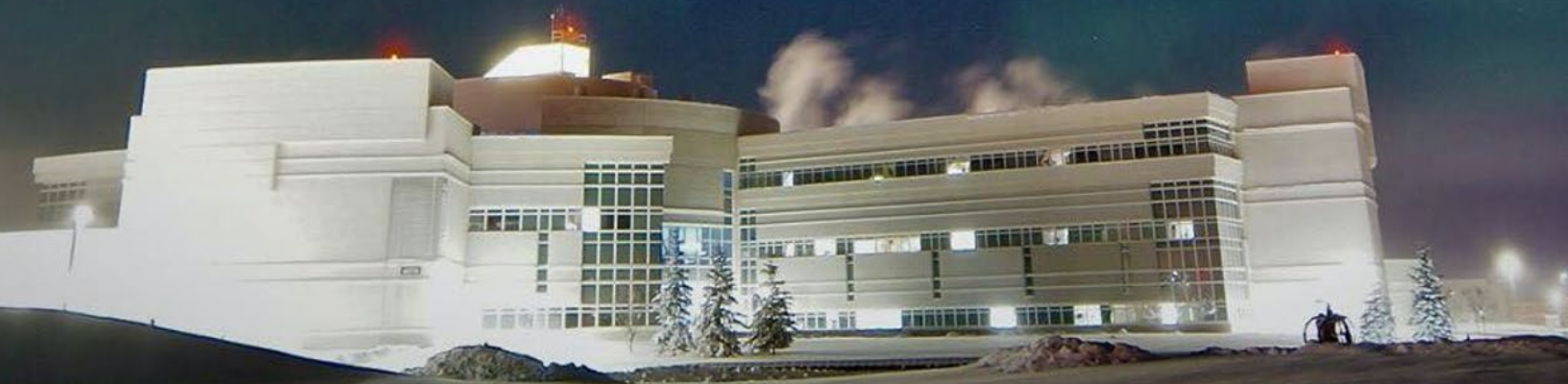
The aurora borealis dances over Bassett Army Community Hospital at Fort Wainwright, AK, as temperatures drop to -20°F. The hospital provides emergency room services and patient care 24 hours a day, 7 days a week.
