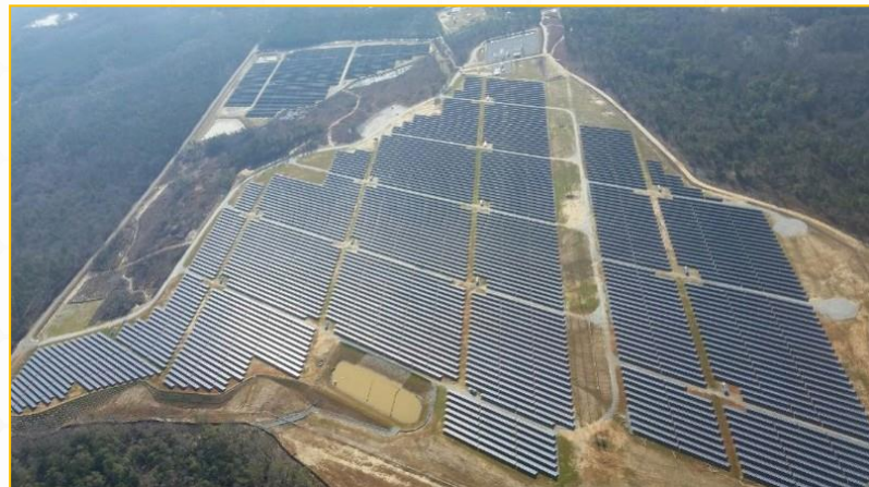
Fort Benning, GA, 30 MW solar array, 133,950 solar panels
