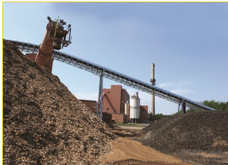
The BGF and intertie provide 100% of the garrison's electricity from a renewable source and includes a 30+ day stockpile of fuel on site.
