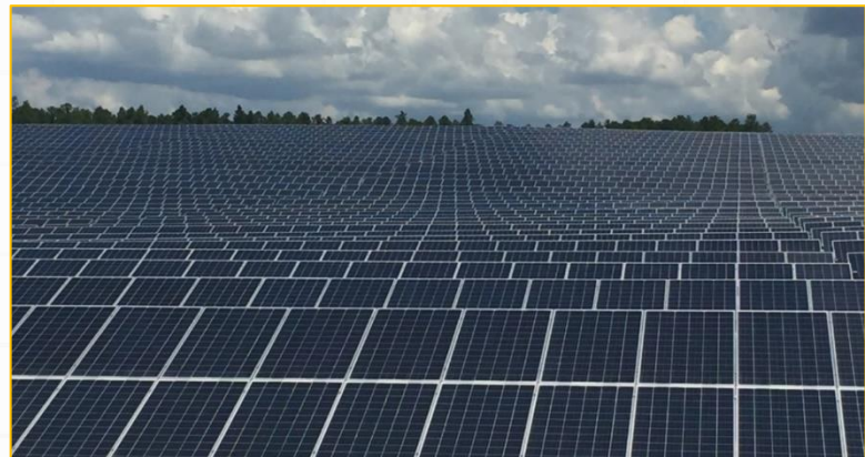
Fort Gordon, GA, 30 MW solar array; 137,520 solar panels.
