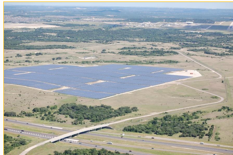
15 MW Onsite Solar Array at Fort Hood, TX
